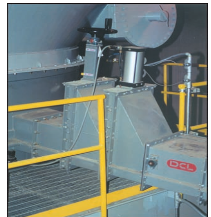
Vertical manual and pneumatic slide gate valve.
