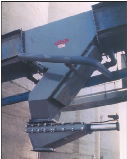
Aerated lump trap with slide gate valve.
