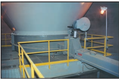
Aerated bin bottom discharging into a conveyor with slide gate valves.
