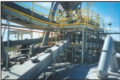
Aeration conveyor run.
