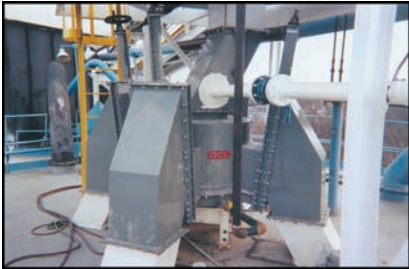
Aerated distribution box with four discharges.
