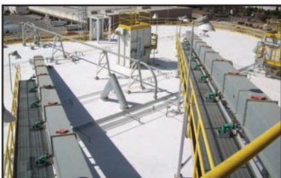
Aeration conveyors feeding multiple silos.
